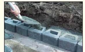
DRAINAGE/BACKFILLING
