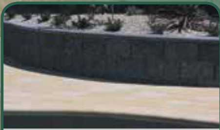
Limestone Bullnose Capping & Classic Stone with Bluestone Tasman Retaining Wall
