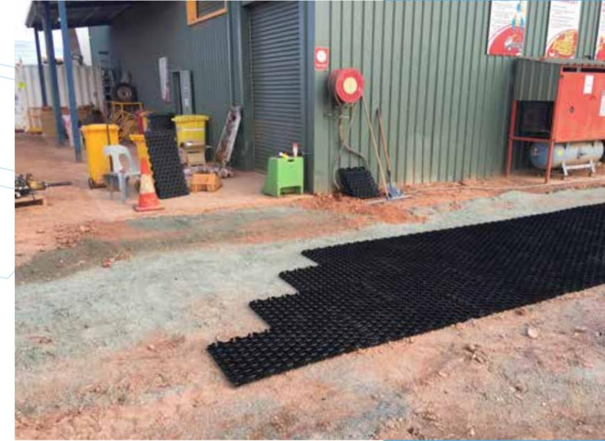
Start point paver, lay first paver with female joining lugs pointing in direction of pavers to be laid
