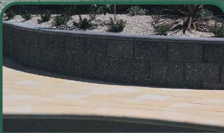
Limestone Bullnose Capping & Classic Stone with Bluestone Freestone Rockface Retaining Wall
